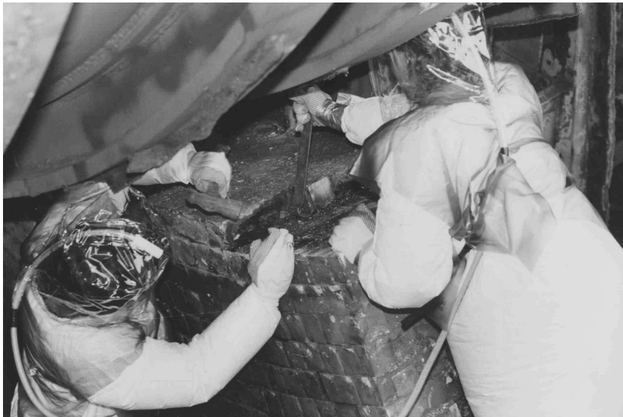
Lead Ballast Removal
