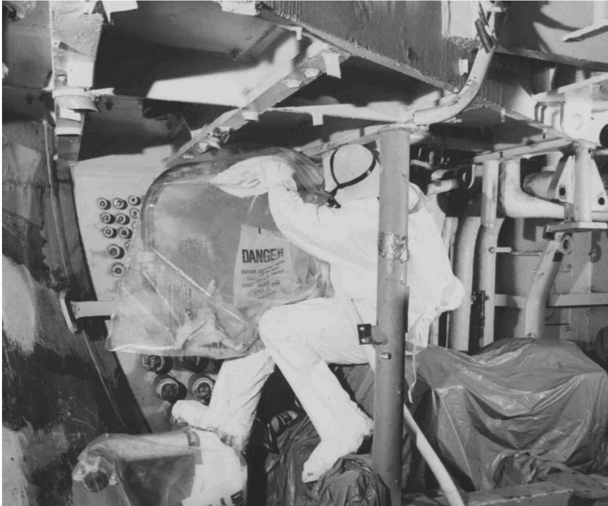
Asbestos Insulation Being Removed from Piping
