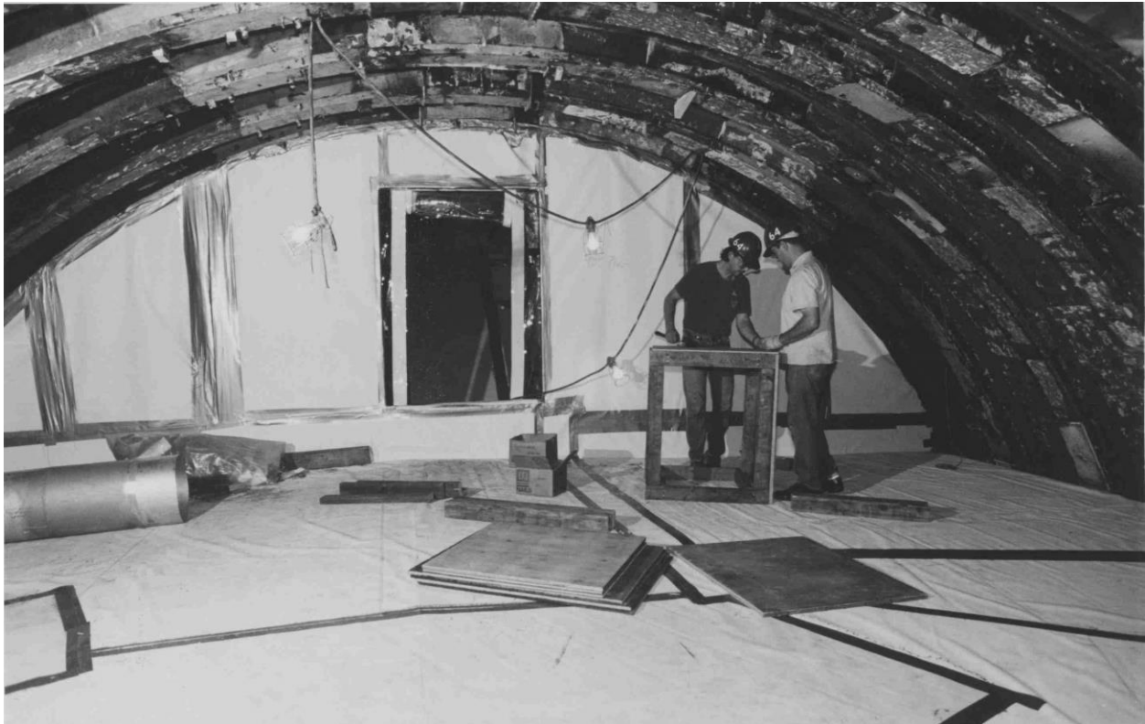
Interior of Submarine with Equipment Removed
