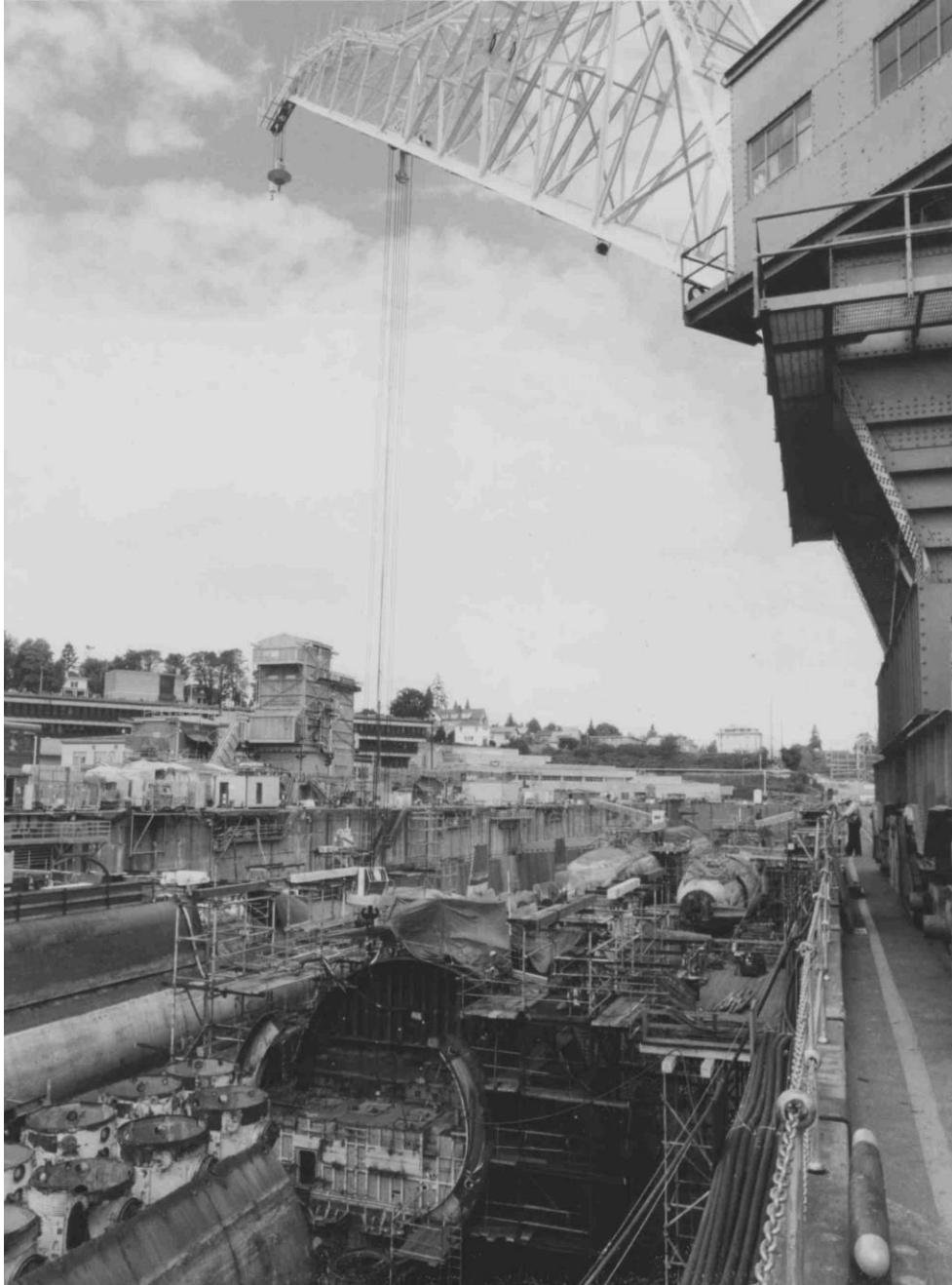
Crane Positioning for Lift of Material from Submarine Undergoing Recycling
