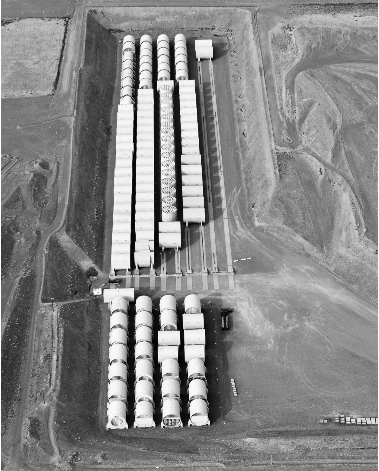
Reactor Compartment Disposal Trench, Fall 2017
