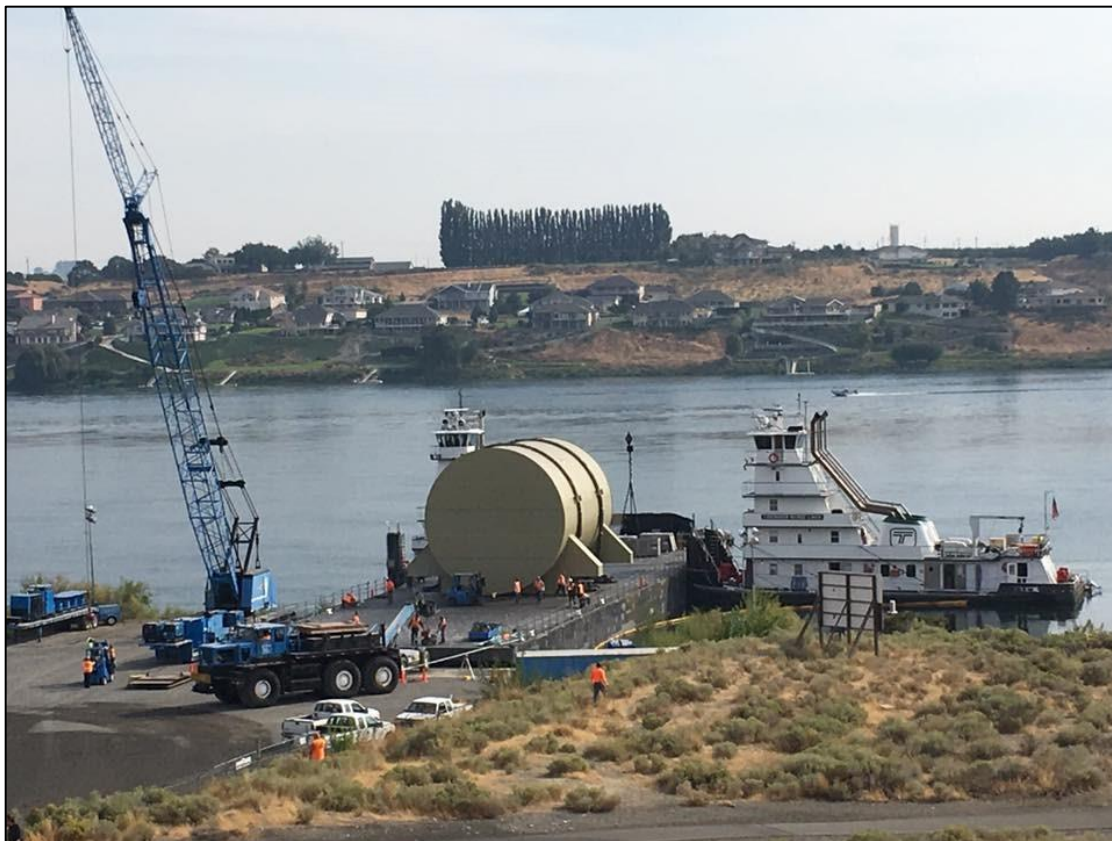
Figure 4. Naval Reactor Compartment Offload in Preparation for Overland Transport to Trench 94, September 2017
